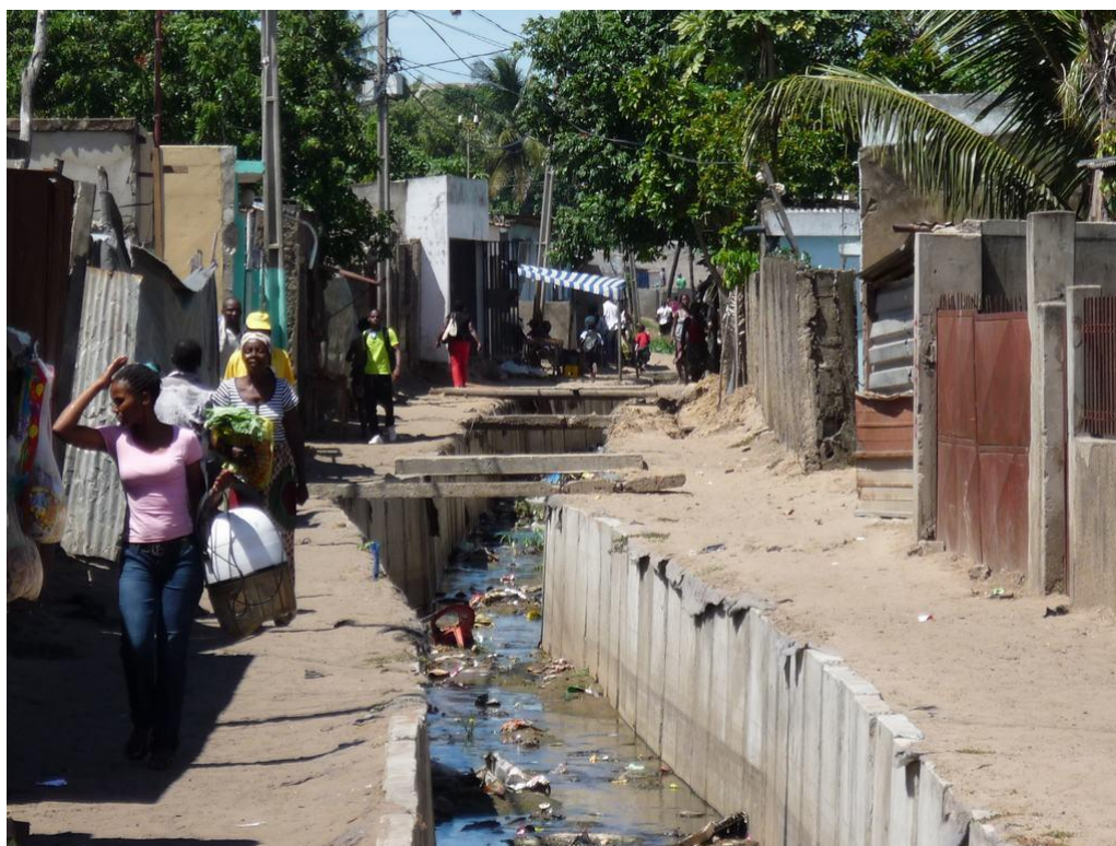
Figure 3-35: Secondary channel in Bairro Maxaquene A, partially filled with solid waste
