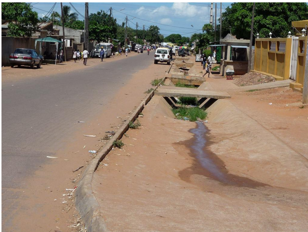
Figure 3-54: Secondary channel in Bairro Sommerschild / Polana Caniço A (close to the detention basin)
