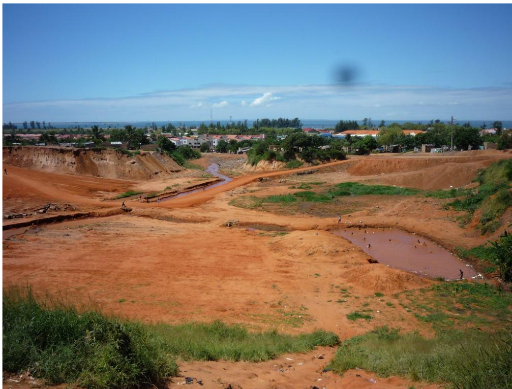
Figure 3-57: Unfinished detention basin North of Sommerschild (at Av. Julius Nyerere)
