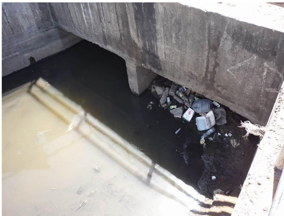
Figure 3-34: Back view of the same culvert
